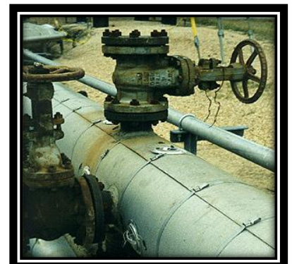
API 570- Pipe Inspection
