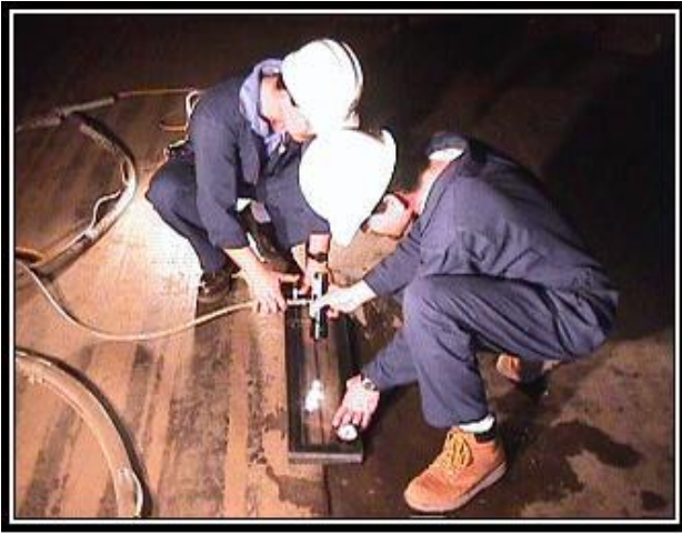
Tank Bottom- Vacuum Box Test
