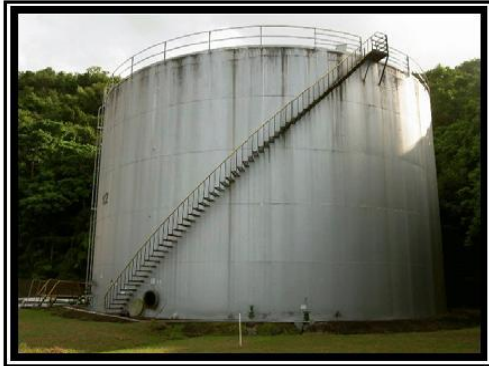
API 653- Tank Inspection
