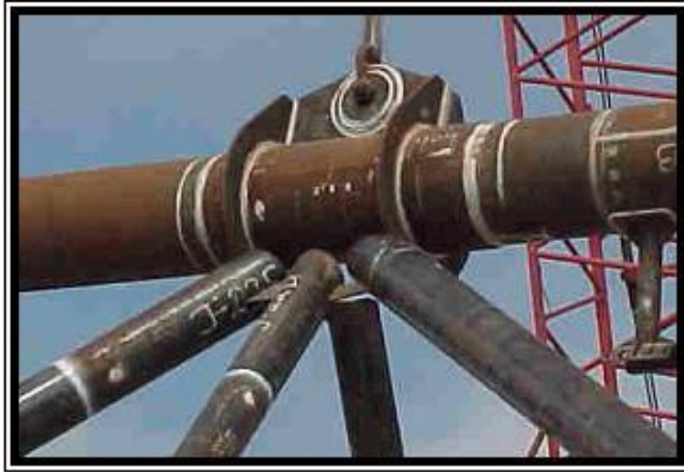
Structural Steel Inspection
